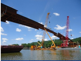
Dick Henderson Bridge, 450-ft river span over navigable waterway requiring coordination with US Coast Guard and US Army Corps of Engineers. Truss removal and new steel girder erection shown.
