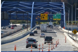
WVDOH Carter Brooks Design-Build Bridge Rehabilitation performed by Kokosing implemented the first ever contra-flow traffic configuration in WV to reduce lane closures.
